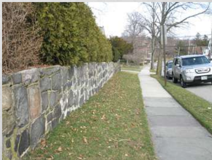
View to the north. Photographed February 2012.
