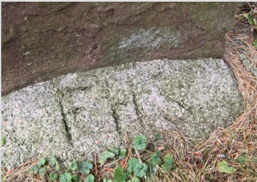
Inscription in concrete at base of marker. Apparently "FHS". Photographed September 2014.
