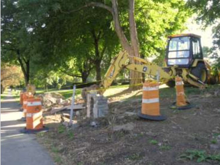
Marker being protected/covered. September 2013.
