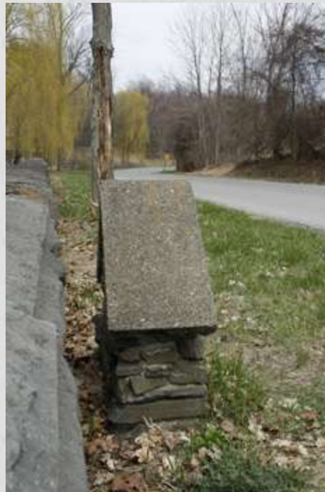
View to the northeast along Old Post Road. Photographed April 2009.
