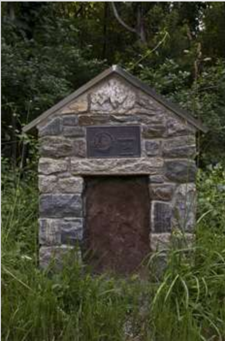
View to the west. Photographed June 2010.
