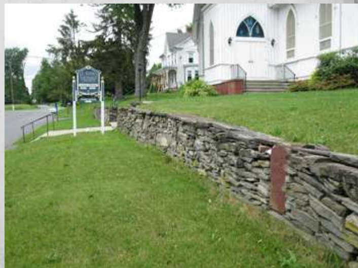
View to the north along Old Post Road North. Photographed June 2011.
