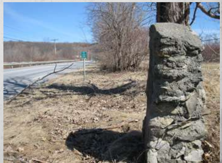
View to the west. Photographed March 2011.
