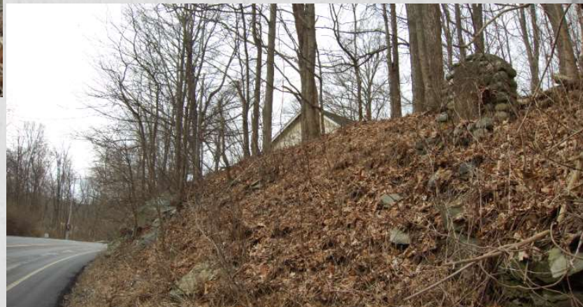
View to the south, January 2019.
