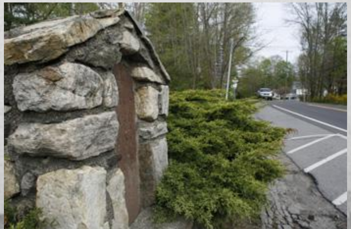
View to the northwest. April 2009.
