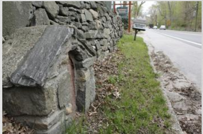
View north. April 2009.
